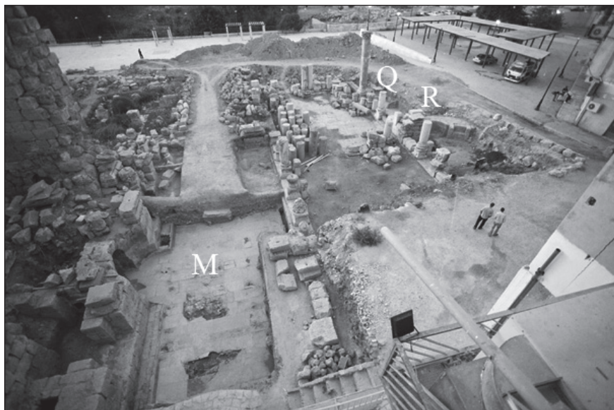
3. Overview of the whole excavation area of the 2017 season.
