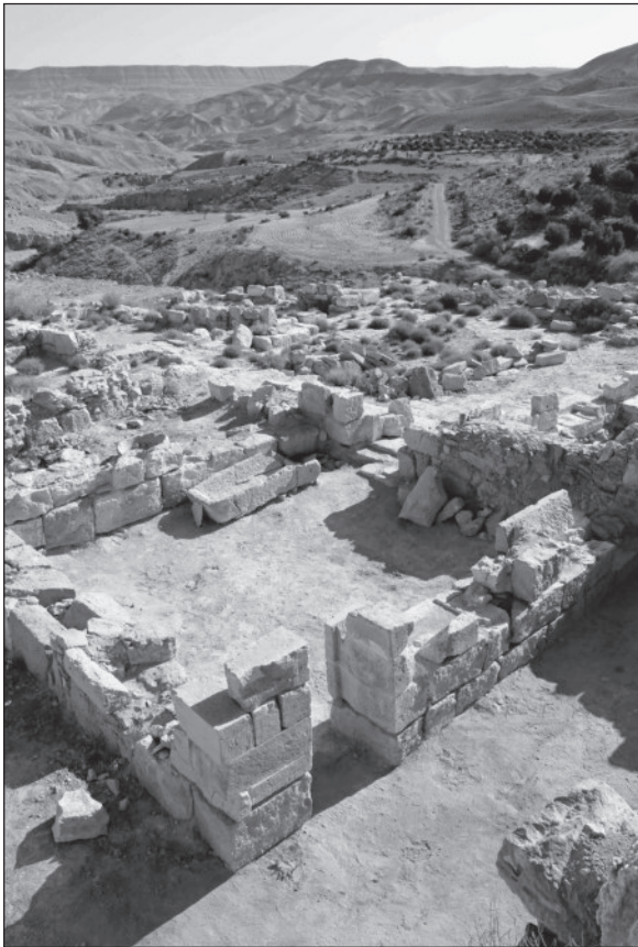
5. Overview of the restored southern wall separating rooms (D) and (E) (© P. P.-F. 2013).
