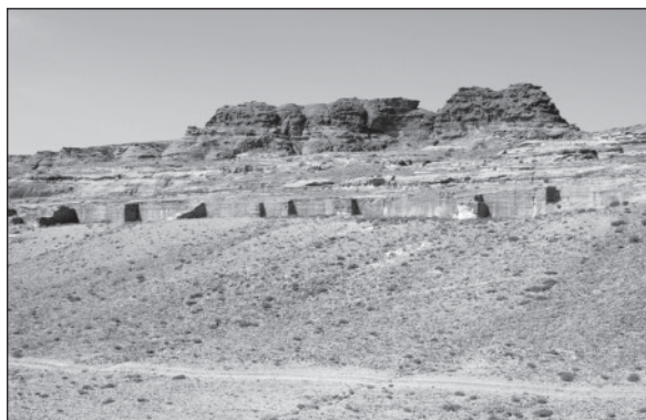
5. R2 Eastern Quarry - Sections 4 - 6 with Wādī al-Burqa in foreground and eastern flanks of Jabal Qalkha in background.
