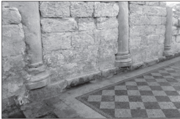
4. Wall D, built on the stylobate, with ashlar filling the intercolumnal spaces and the mosaic flooring of Passage C in Square E108. (Photo: the author, 2014).
