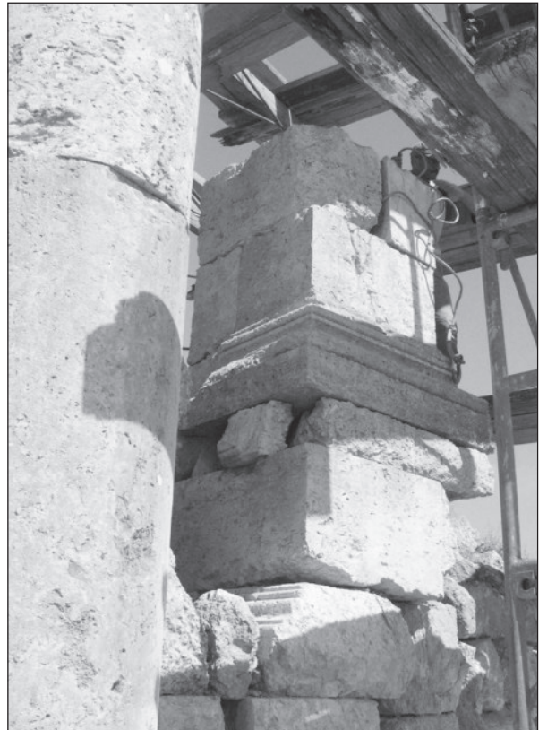
5. North-west pillar in antis during dismantling, from the south-east.
