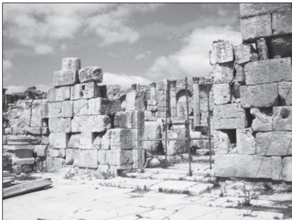
12. West wall of the Propylaea Church in 2009, from the north-west.
