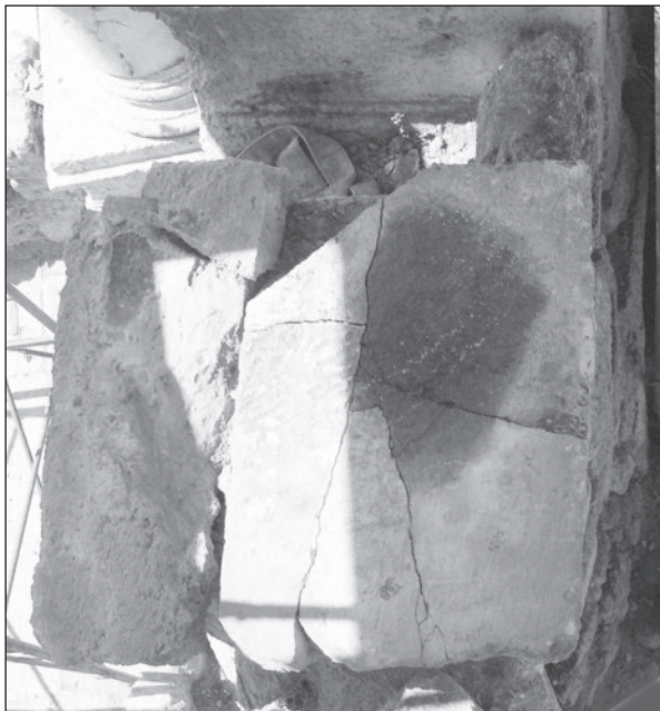
6. North-west pillar in antis ; upper cornice of the plinth during dismantling, from above.
