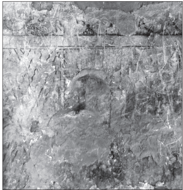
31. The faux marble area (before conservation).
