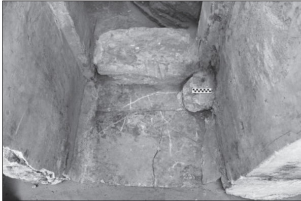
6. Door jamb and post with copper hinge in doorway between tepidarium and frigidarium .
