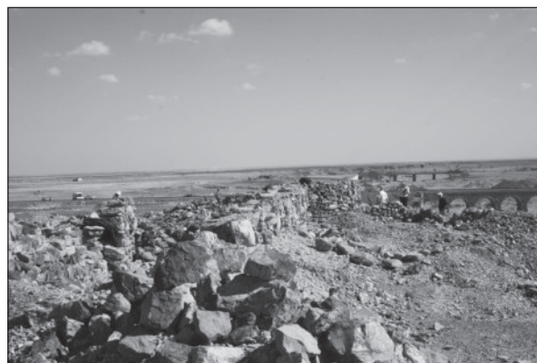
4. Mākīn’s Fort with viaduct in background (copyright GARP).
