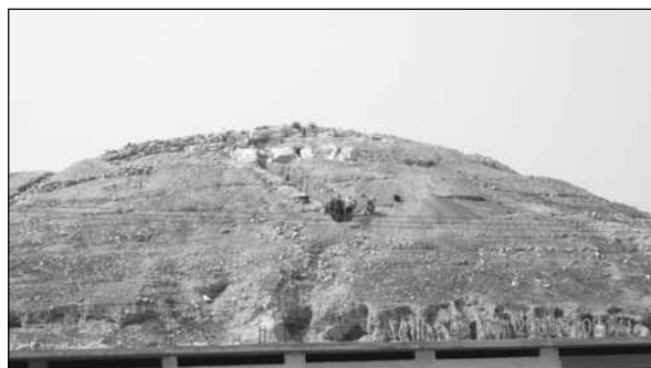
20. Exploratory trench: view from north.
