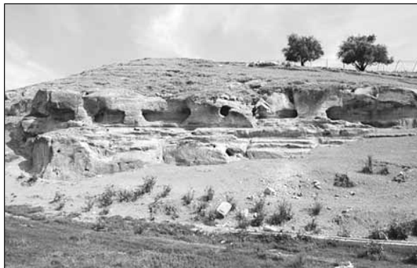
11. Rock-cut tunnel aqueduct, site 666.
