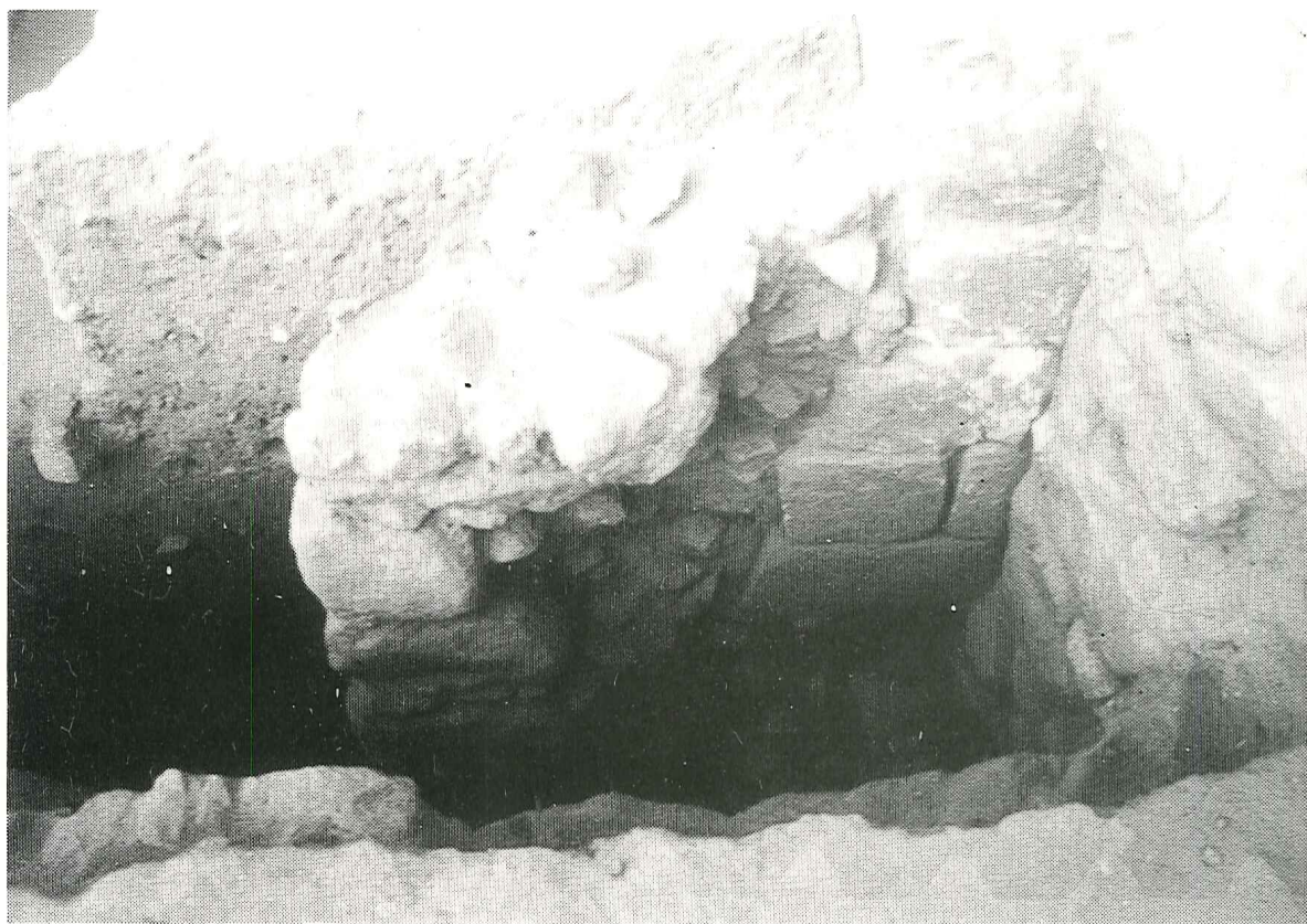
2. Wall D13c-K, displacement of northeast face.
