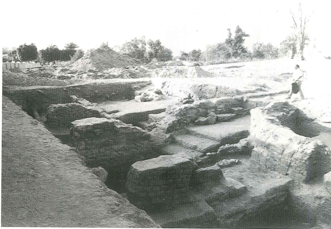
1. Area F, looking to the south.
