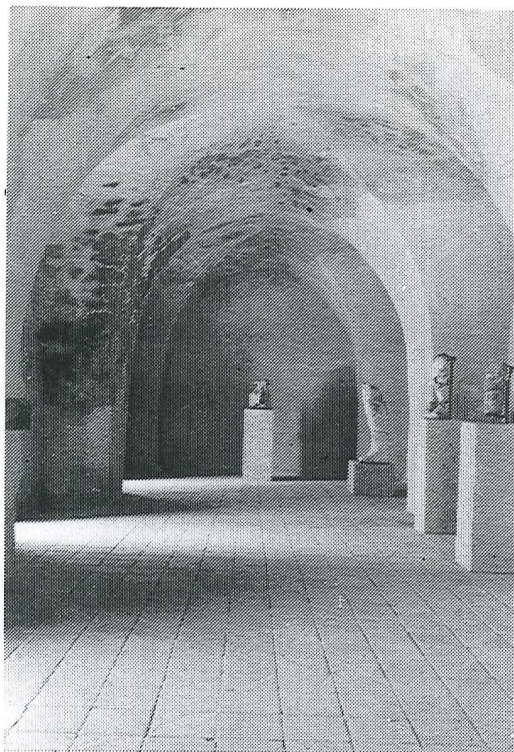
1. Umm Qeis, Beit ar-Rusan (Museum): Cross-vaulted exhibition hall for the collection of Roman marble sculpture, situation October 1990.
