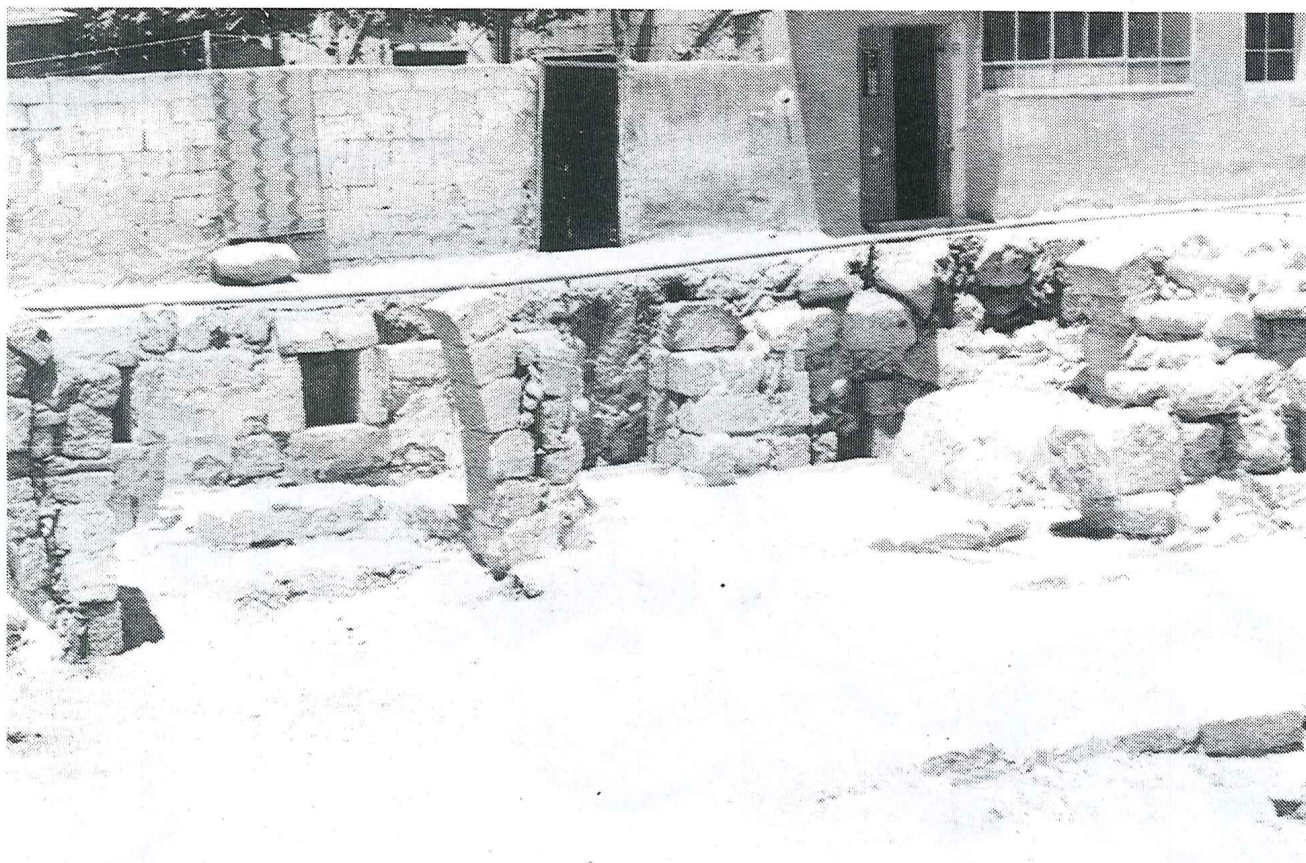
2. View to west of west central and northwest rooms.
