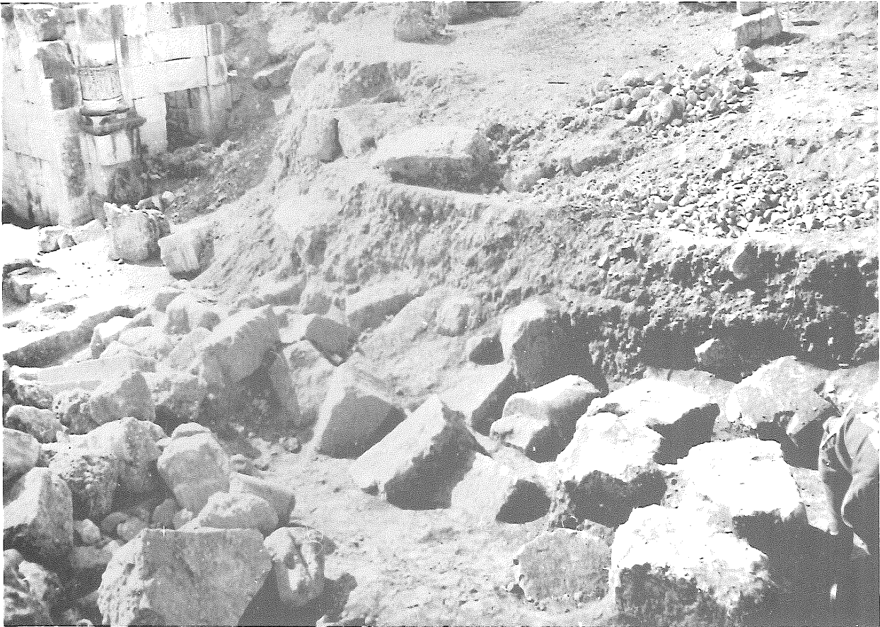
Pl. LXXXIX, 1 - Elements of South Pavillon as they have fallen.
