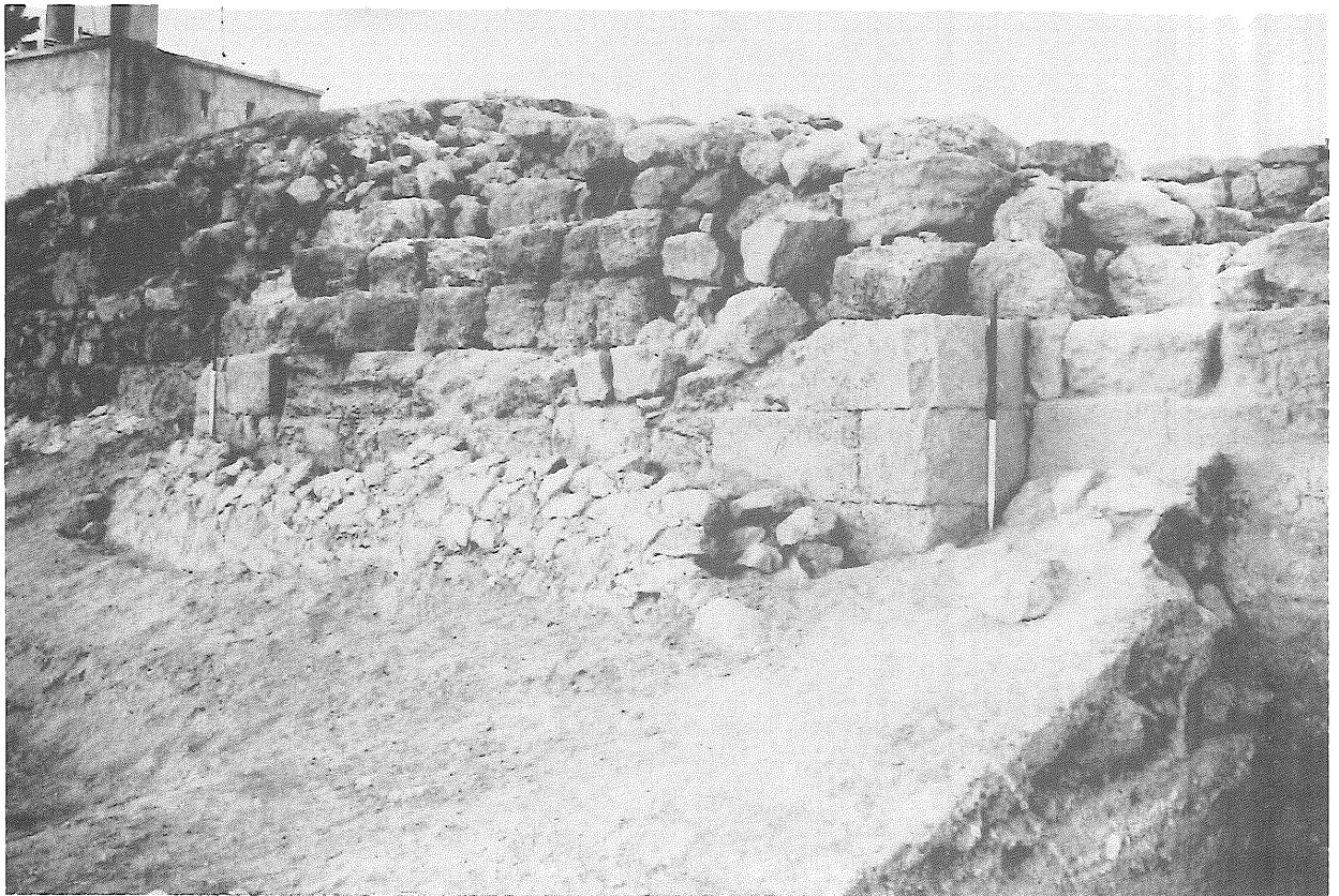
Pl. XCVIII,2-Umayyad defensive wall showing different phases, looking E.
