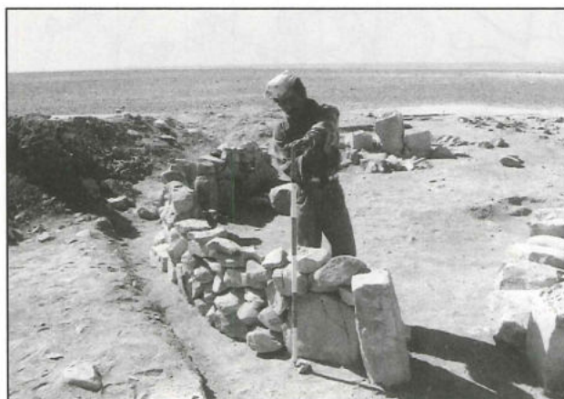
5. Structure 07: an experimental reconstruction of the southern wall.
