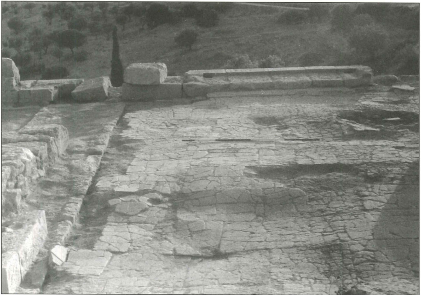
4 .Umm Qays, Area I. The Terrace's west retaining wall with basalt doorsill; southern perimeter wall (looking W).
