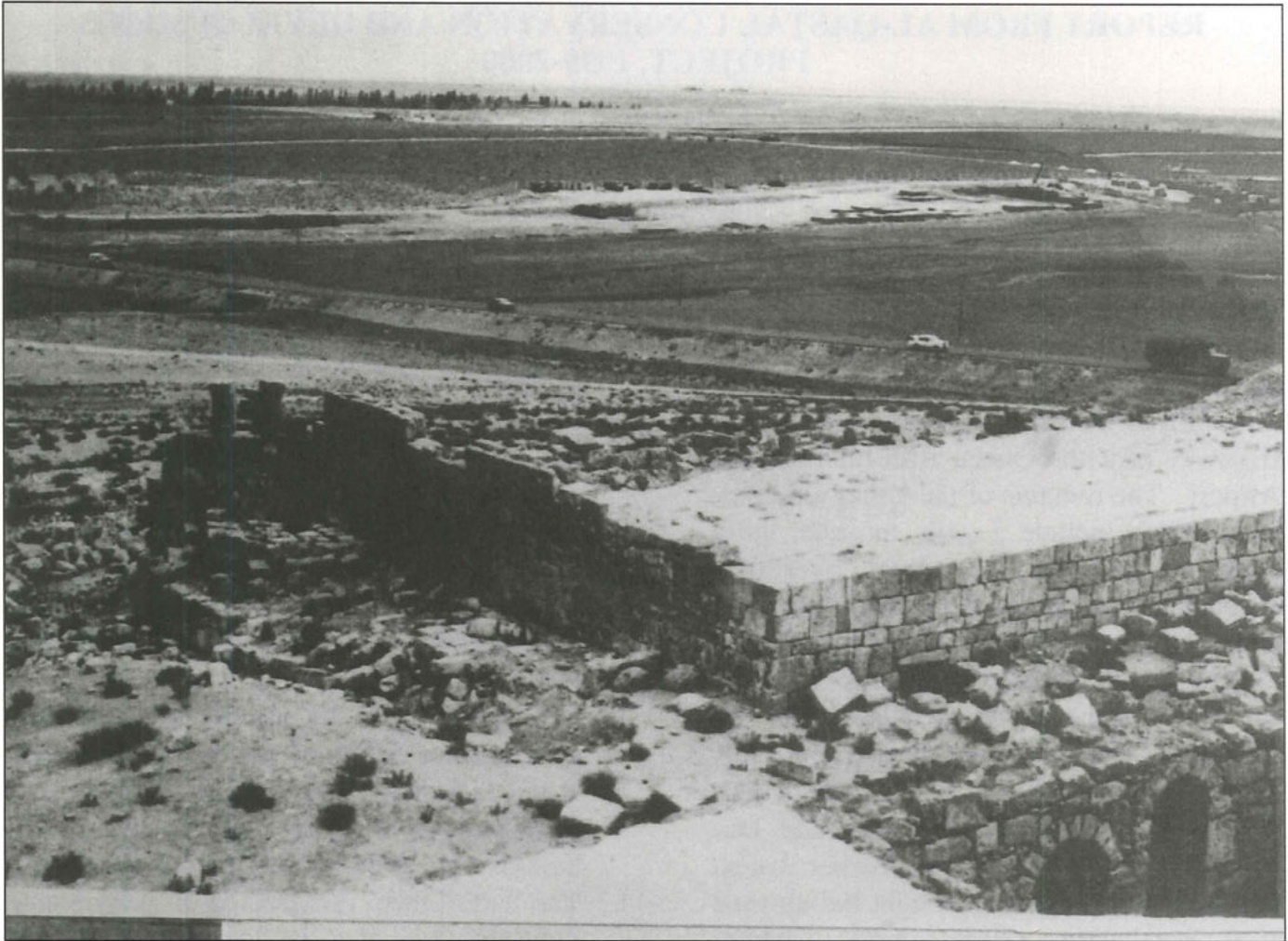
1. View of mosque from southwest (DAJ archives/ late 1960s), before the expansion of dīwān Shibli al-Fayez. Note the two arched doorways in the extreme lower right foreground: referred to as “shops” by al-Qaṣṭal locals. Dates for Figs. 1 and 4-6 are determined by the presence or absence of the orchard barely visible in the upper left corner of Fig. 1, and clearly visible in the background of Fig. 6.
