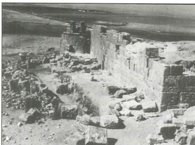
5. Southwest corner of mosque (DAJ archives, 1960s). Again, where the southwest corner of the enclosure walls has collapsed, only earth is visible inside.
