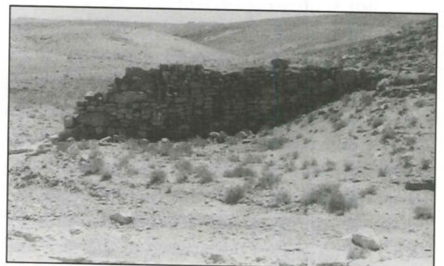
2. A Potential Nabataean Dam (Site 223) at the Wādī al-Qaṭṭar.
