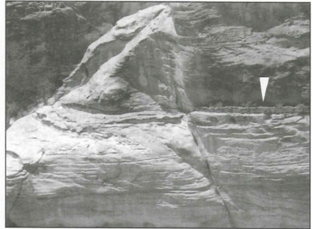
22. Rock-cut and built Conduit at the southern cliff of Wādi Mūsā.
