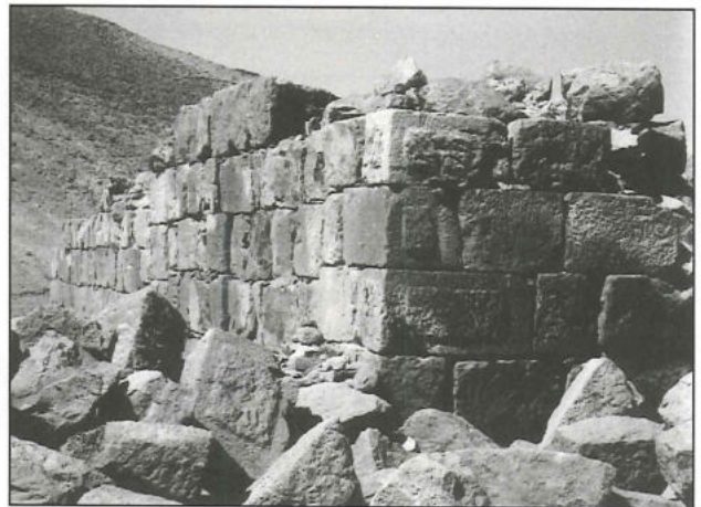
13. Older Part of Qaşr Umm Ratam with bossed cornerstones and a crenel.
