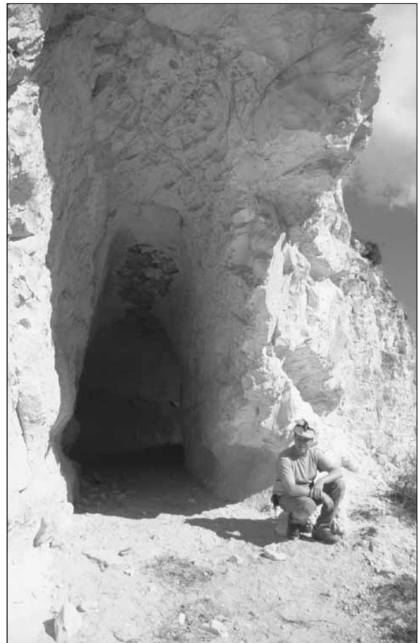
15. A landslide caused by tunnel construction exposed the route in Wādī ash-Shallālah.
