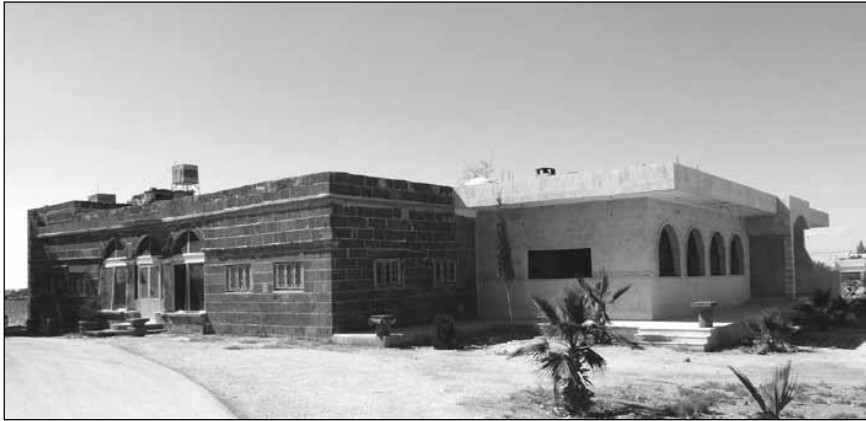
3. House built by Shaykh Hail es-Serour showing old and new construction (aesthetic/status model). The original basalt house built in the 1960s is on the left and the madhafa addition, which replaced the majlis tent in the 1990s, is on the right. Monumental architectural fragments are visible on the porches (photo by Bert de Vries).
