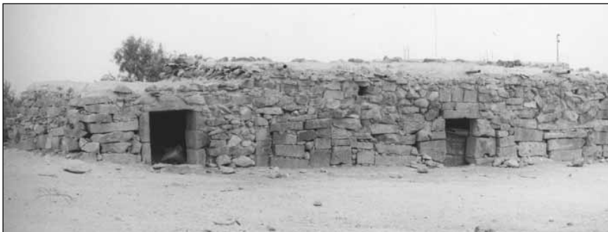
4. Older, poorer home to the east of Umm al-Jimāl, now used for storage, constructed of stone rubble and spoiled blocks taken as free building material (utilitarian model) (photo by Janet Brashler).
