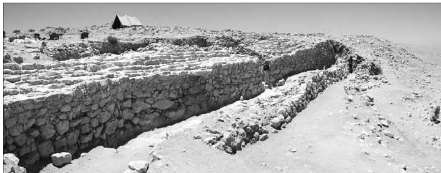
7. The EB IIIA double line of fortifications, with EB II - III main city wall to left and parallel outer wall W.155 to right, from north-east.
