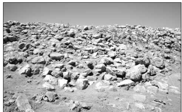
4. The EB IV embankment, from north-east.
