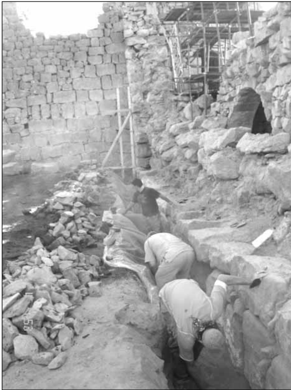
5. Wall 22 after dismantling (foundation preservation process).
