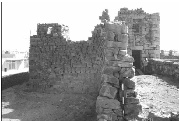
2. Wall 22 before reconstruction (looking to north from the top).
