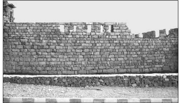
6. Wall 22 after reconstruction (looking to east).
