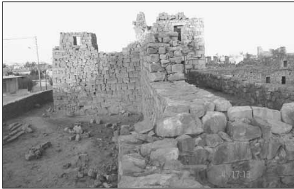
8. Wall 22 after reconstruction (looking north from the top).
