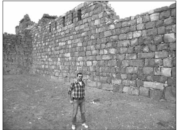
7. Wall 22 after reconstruction (looking to north).
