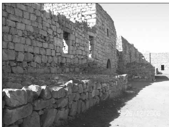
11. courtyard before excavation (looking S.W.).
