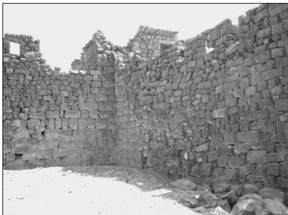
3. Wall 22 before reconstruction (looking to north).
