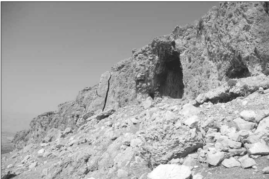
5. Mughr al-Ḥamāmah 2 looking east, with rockfall-strewn terrace in the foreground. Massive roof collapse indicates a former outer chamber, which is now collapsed.
