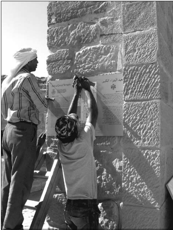
9. Sign installation, 2007 (Artemis W. Joukowsky).
