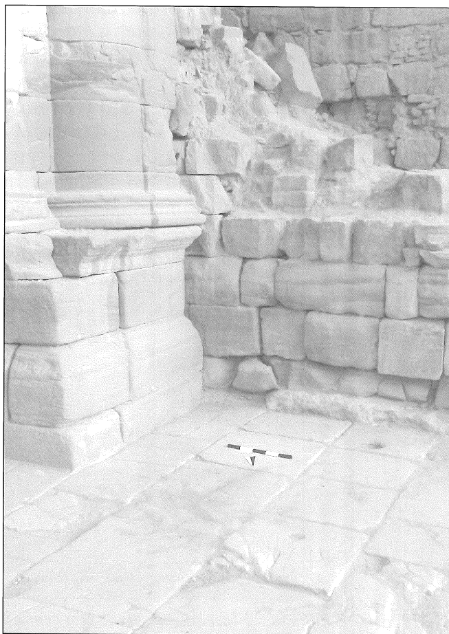
24. Trench 4 after excavation (Schmid).
