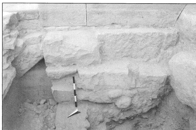
9. Trench 4, foundation of the Temenos Gate after cleaning (Schmid).
