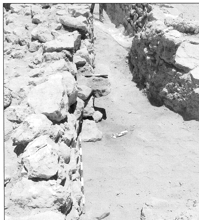
9. The inner staircase (W.181), which led to the top of the EB III main city-wall W.105c-b, from west.
