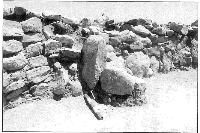
8. Unit 03 of Complex I: a buttress attached to the eastern wall (from NW).
