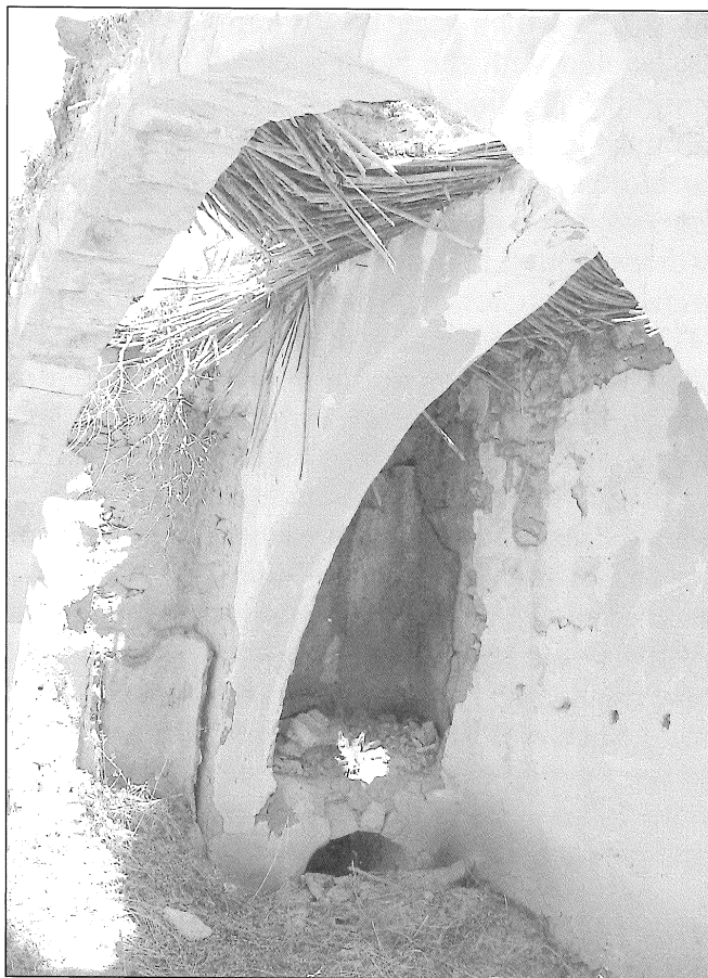
20. Interior of 'Obeidat farmhouse, illustrating transverse arch forms of construction.
