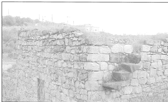
18. Staircase of Mandate-period mosque at Ḥubrāṣ, built into the outer face of the qibla wall, rebuilt in 1931 "Prayers were done from the roof."
