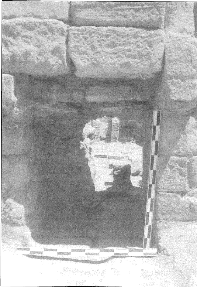
16. Communicating passage between the caldaria.
