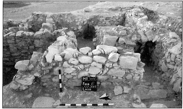
11. Field B, Pillared Building 205, looking east, with arched doorway on the right, attached to W2022.
