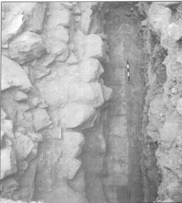
19. The northern foundation of the staircase running east-west and built with yellow limestone blocks over natural rock.
