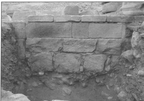
25. Trench 2, foundation trench of Nabataean wall partially excavated (Schmid).
