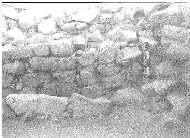
10. Photo of Square I3's blocked doorway (32) in Walls 23 and 33 (left = west of scale stick); view to the north.
