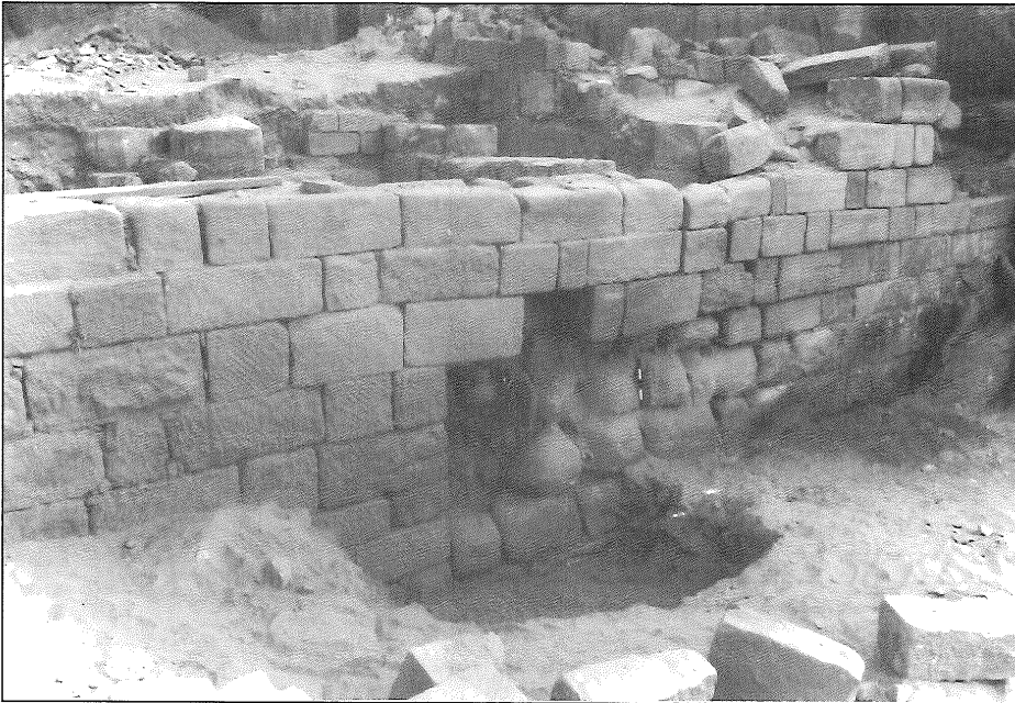
9. Lower terrace, main retaining wall of the lower terrace from N, showing the original part on the left, later additions on the right (Schmid).
