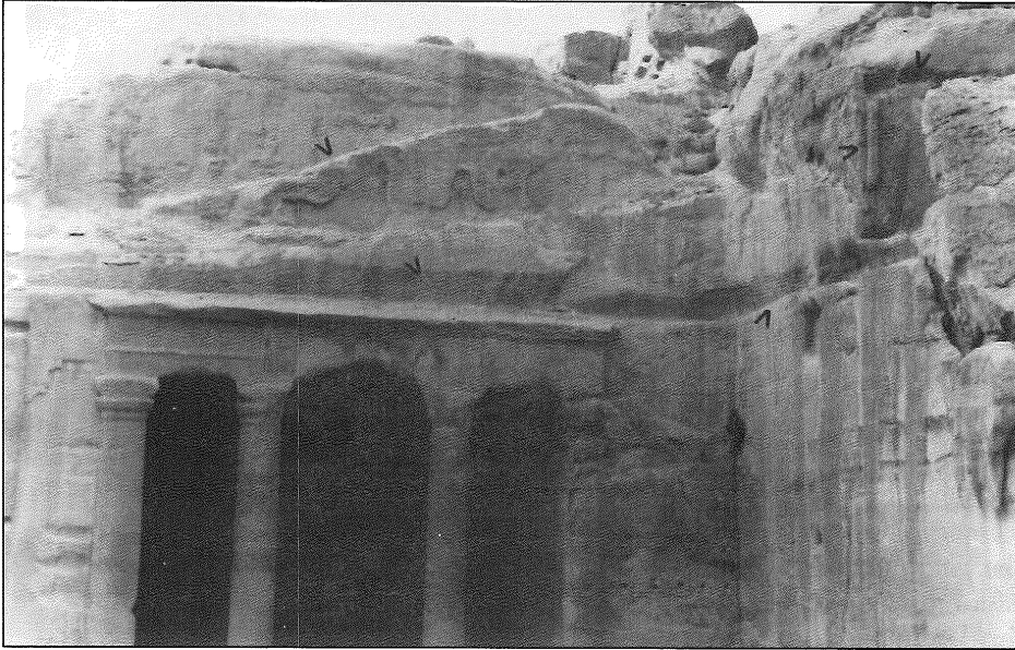
37. Upper terrace, "Garden Triclinium" and related structures (rock-cuttings for upper floor etc.) from S (Schmid).
