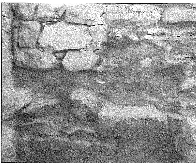
7. Consolidated mud mortar of Wall G in Trench O after treatment (by J. Latikka).
