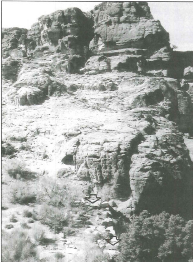
15. Dam, 17m long, 4.30m wide and 5.30 high some 100m above Wādī Šabrā (arrow) (1987).
