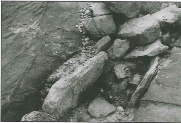
20. Re-used section of the northern conduit of Ba'ja I (1986).
