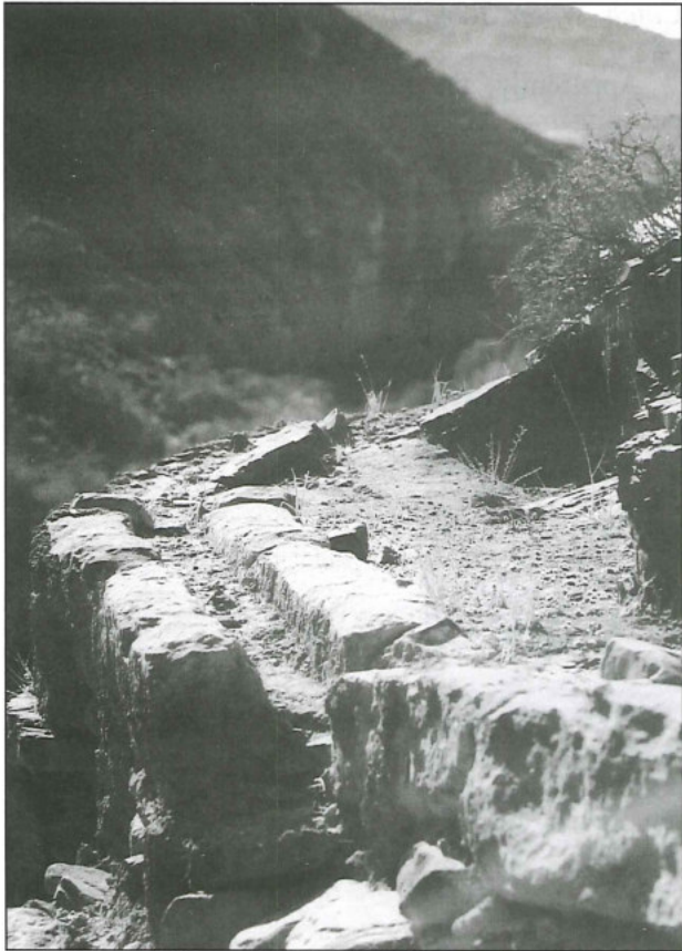
8. Prefabricated conduit blocks at the quartz-porphry wall high above the wadi (1988).
