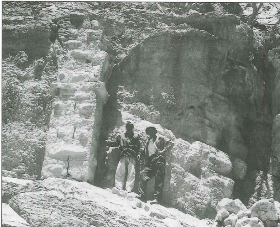
12. Broken-down aqueduct arch (2003).
