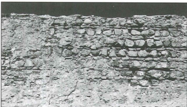
3. Al-Ḥammām, detail of the cistern's masonry (photo D. Genequand).
