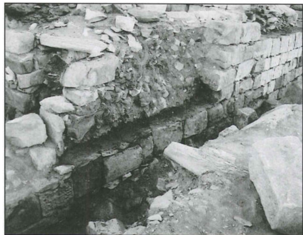
13. Wall supporting the apse, before the restoration (by Ch. Danielli).
