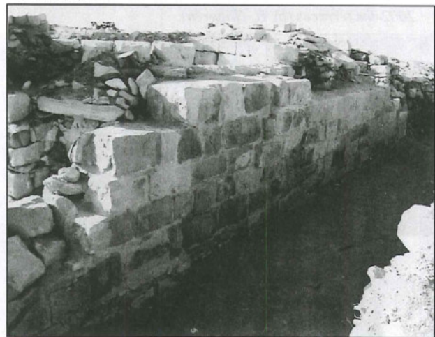
14. Wall supporting the apse, after the restoration (by Ch. Danielli).
