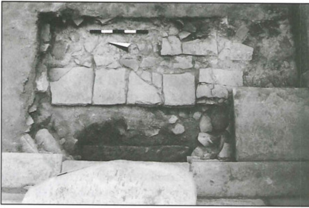
3. Lower terrace, S-corner of room 1 with floor slabs and sa-maga-foundation (Schmid).
