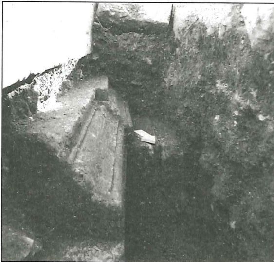
3. Jarash, Cathedral. moulding under the eastern walk of the atrium.
