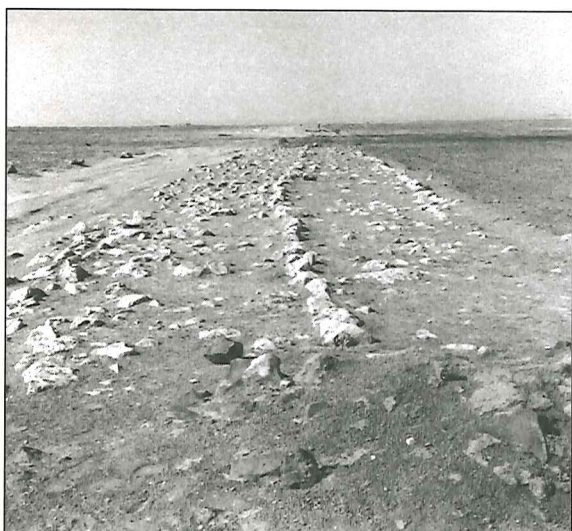
3. The same view of the Via Nova Traiana west of Umm al-Jimāl in 1978. NB ploughing was far less encroaching.
