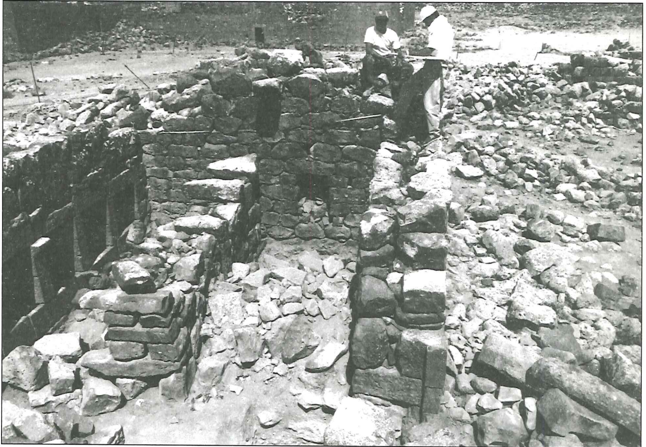
4. Stable A with architect al-Bataineh recording its masonry. The wall with the mangers is on the left and the Drüz wall intended as filler for the erection of an arch in the center.(Photo by B. de Vries).
