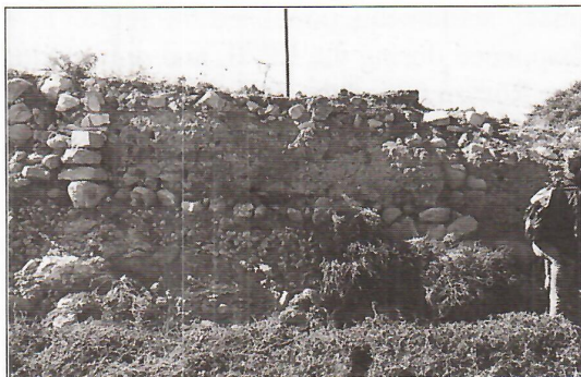
6: Site 79: EBII remains of mudbrick structures on stone foundations, visible in a bulldozer cut.
