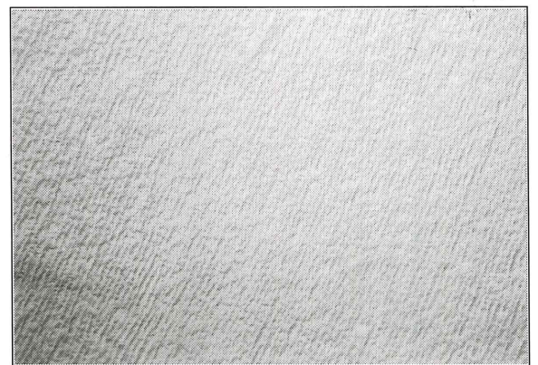
18. Diagonal dressing of the stone.
