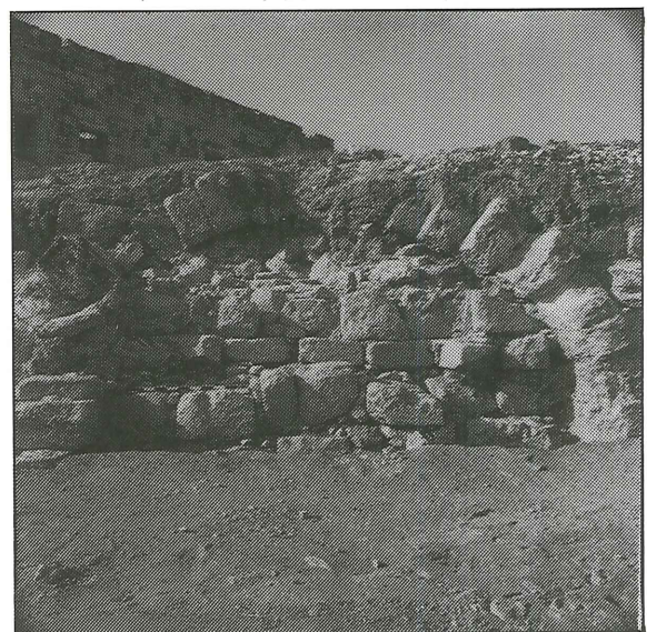
3. Area 3-5: Last arch of the aqueduct .
