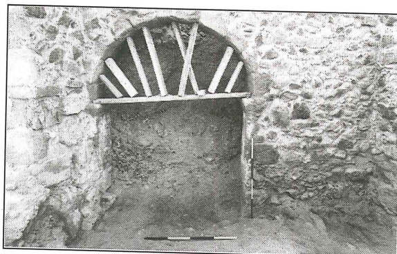
9. Supporting arch under north aisle of church, F. I 4.1/H. II 7 (Photo T. Springett).
