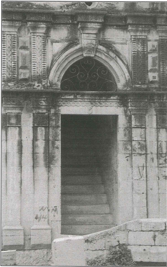
8. Main portal of the Bayt Abujaber.
