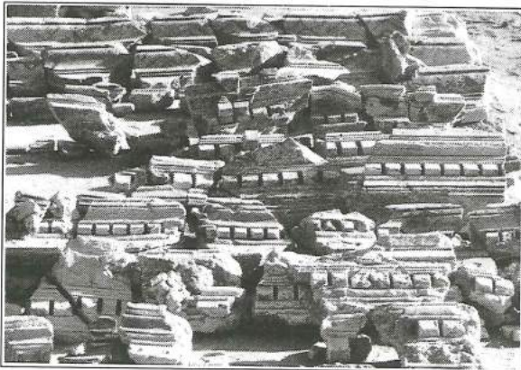
7. EZ IV. View of fragmented stucco cornices from room 6 (photo: O. Jäggi).
