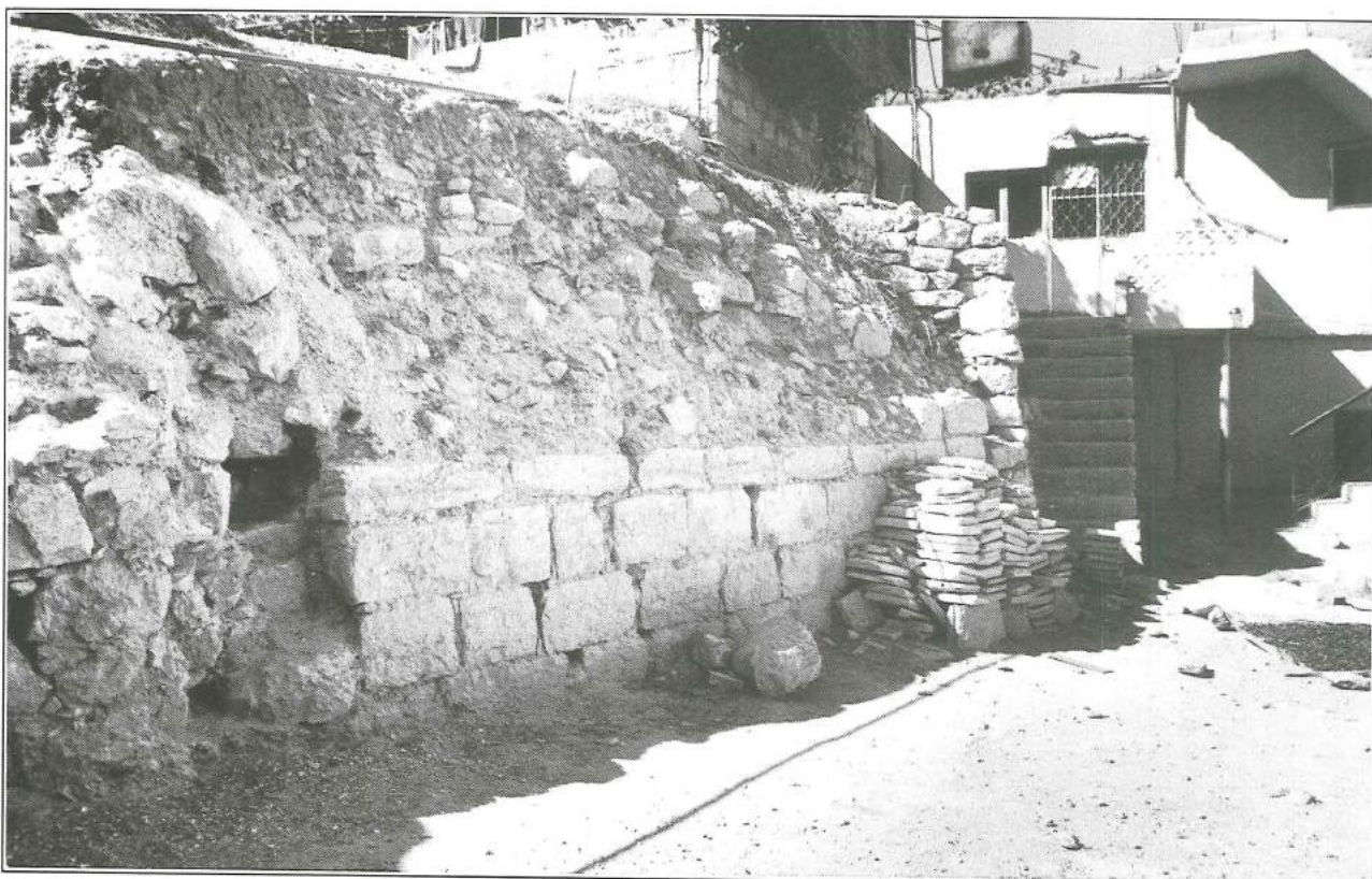
15. WMS 1996 site Wadi Musa 18J: ancient wall preserved at the back of a modern courtyard.
