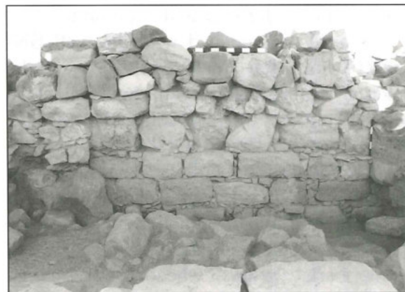
18. Wall in N-9 showing secondary rebuild; view toward west.
