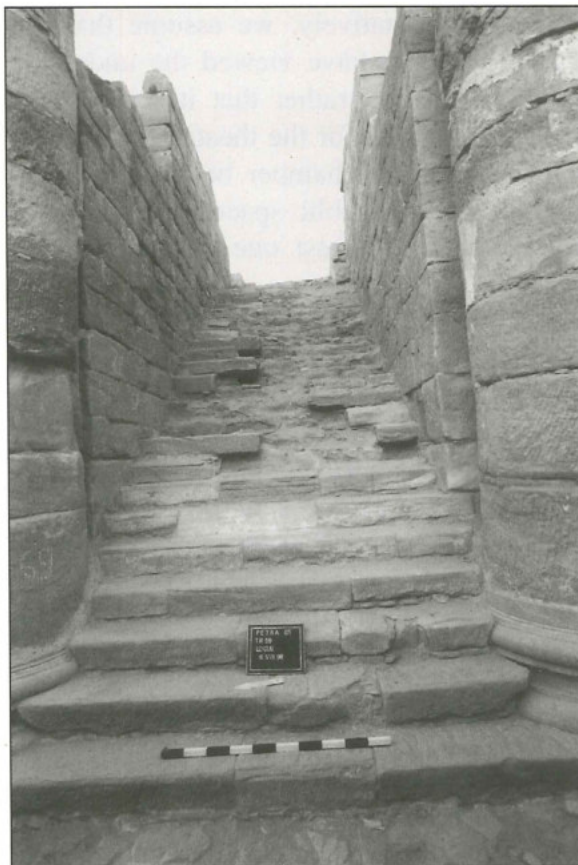
25. 1998, Southwest Stairway extending down to the West Corridor, before conservation (Artemis A. W. Joukowsky).
