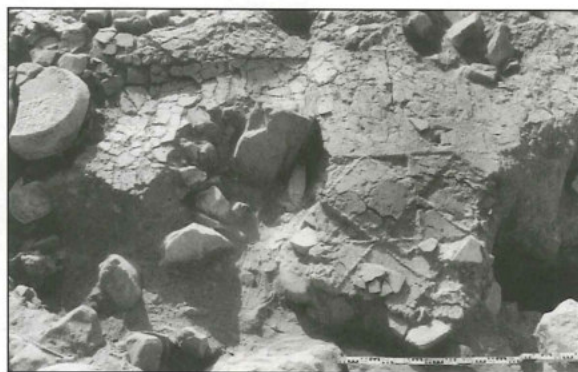
4. EZ IV, room 17. Mortar bedding of opus sectile pavement with fragments of marble tiles. (photo: D. Keller).
