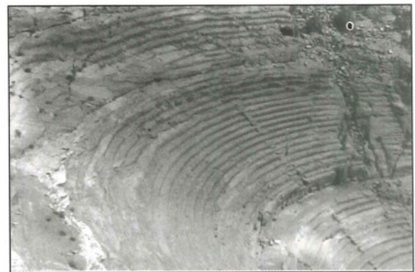
6. The recessed surfaces were measured from the ima cavea and media cavea of the Theater. The enclosed nature of the Roman Theater in the Outer as-Siq of Petra permits the seasonal balance between a weathering-limited (winter) and erosion-limited (summer) environments.
